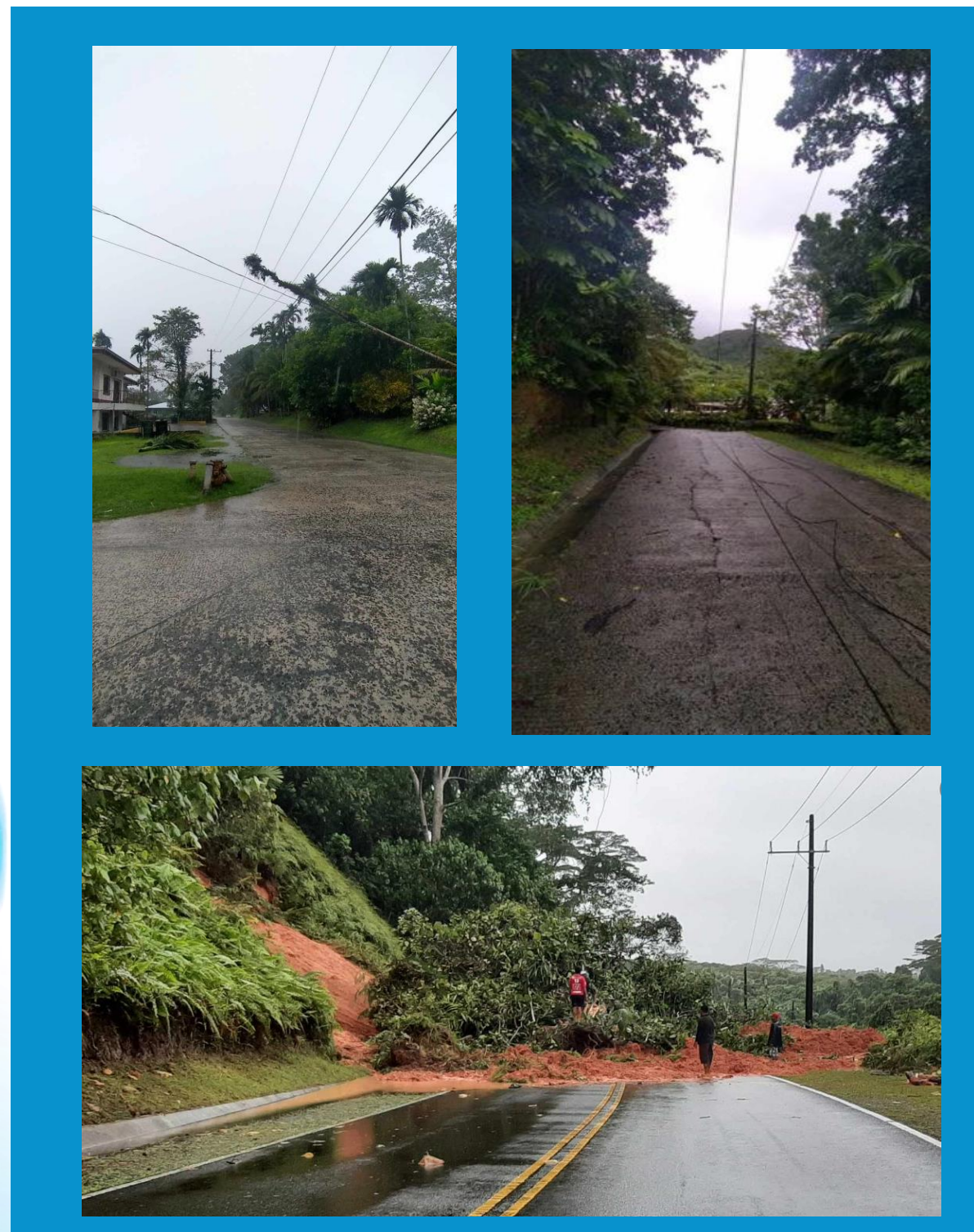
Fallen tree damaging power lines and hardware in Ngermid and Aimeliik on Sep. 11, 2024. Credits: PPUC Significant landslide at Ngarmeskang, Ngeremlengui on Sep. 12, 2024. Credits: Ngeremlengui State
