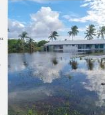
Tetautua Primary School in Penrhyn pictured at 7.30am yesterday, was surrounded by sea water. PC: TAMU TAPU/TAU/24020501
