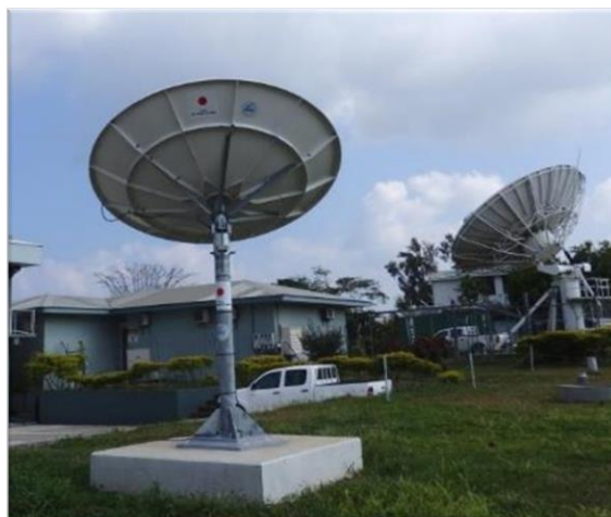
HimawariCast receiving system in Vanuatu
